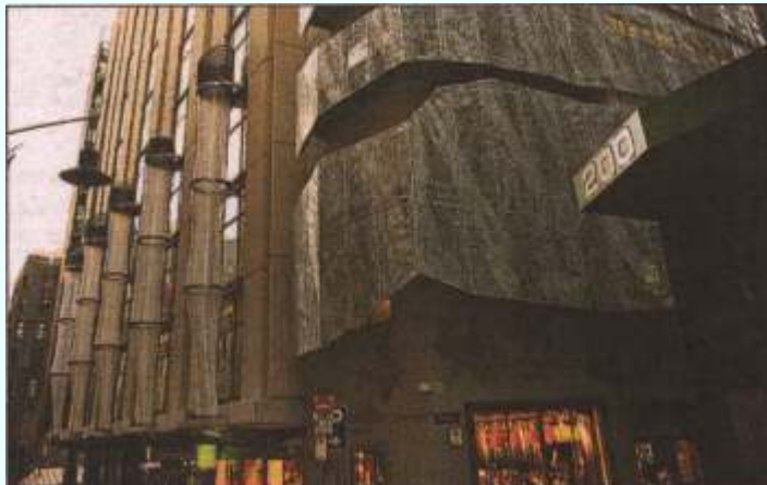
The CH2 building has set zero net emissions by 2020. Photo: JOHN WOULDSTRA
