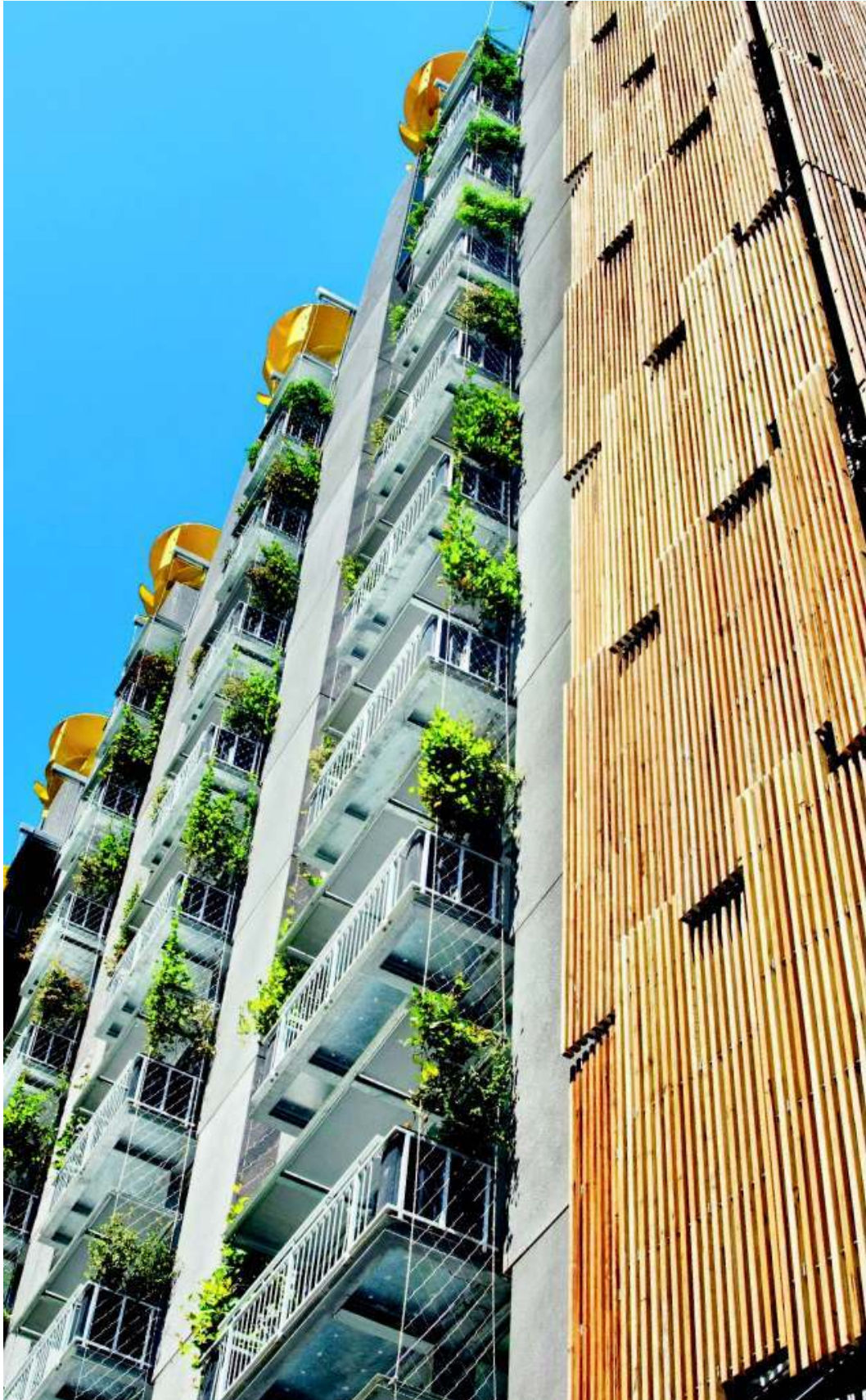
The timber louvres shade the western facade of Council House 2 and move according to the position of the sun
