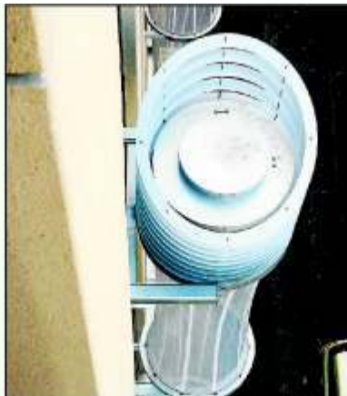
A shower tower cools air with water
